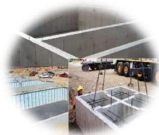
Cast off site Prefabrication
