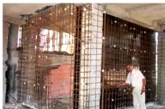
Addition of Shear Walls
