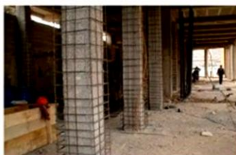
Jacketing of columns
