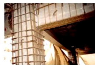
Beam column joint jacking
