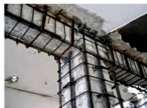
Jacketing of beams
