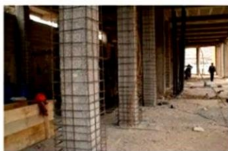
Jacketing of columns
