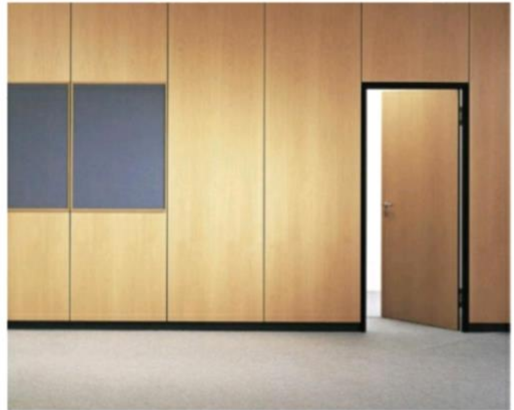
Wooden partition wall
