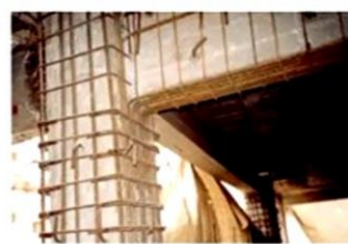
Beam column joint jacking
