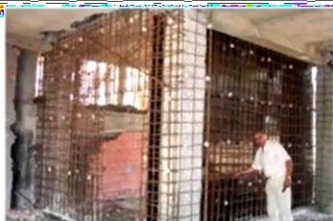
Addition of Shear Walls
