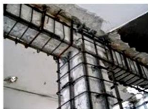
Jacketing of beams
