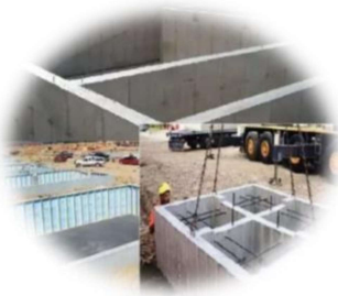
Cast off site Prefabrication
